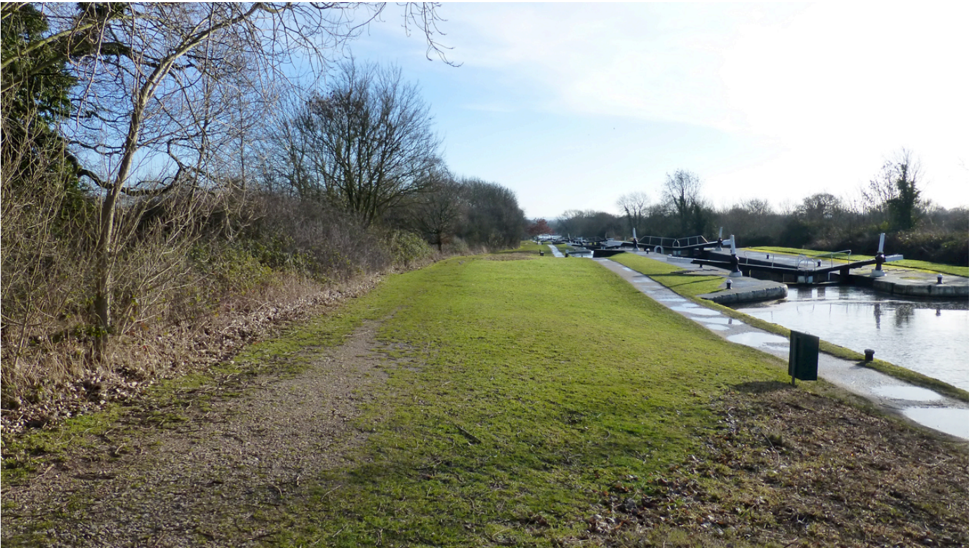
Photo 1 – View along canal corridor contained by adjacent vegetation
