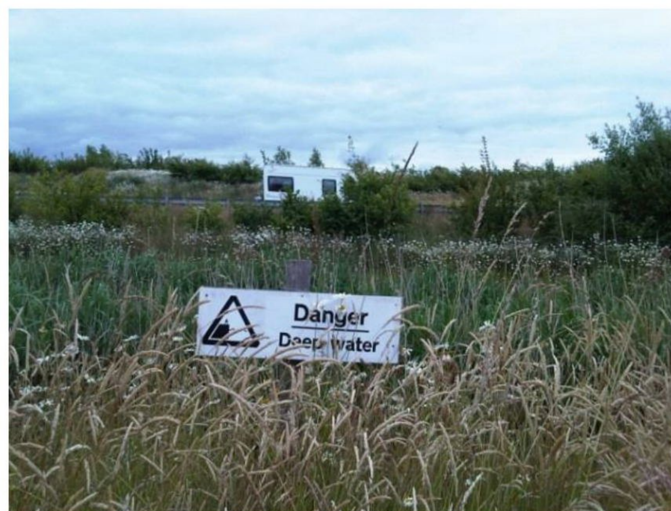
Drainage ponds actually within GT12. Bypass in the background.
