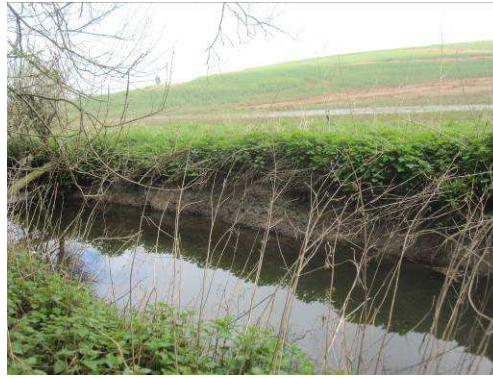
Sheer earth bank on Tach Brook with potential for kingfisher holes.
