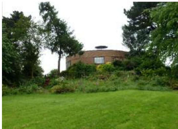
Existing residential properties adjacent to the golf course
