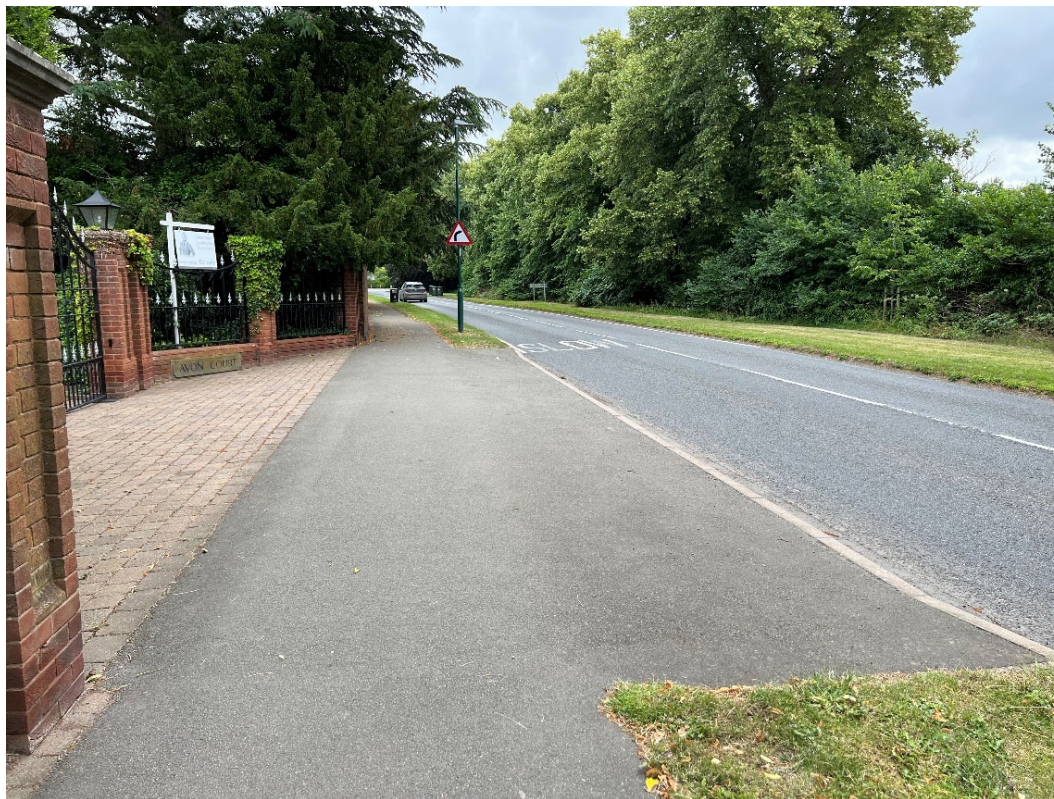
Photo 1 - Existing Footway Main Street
