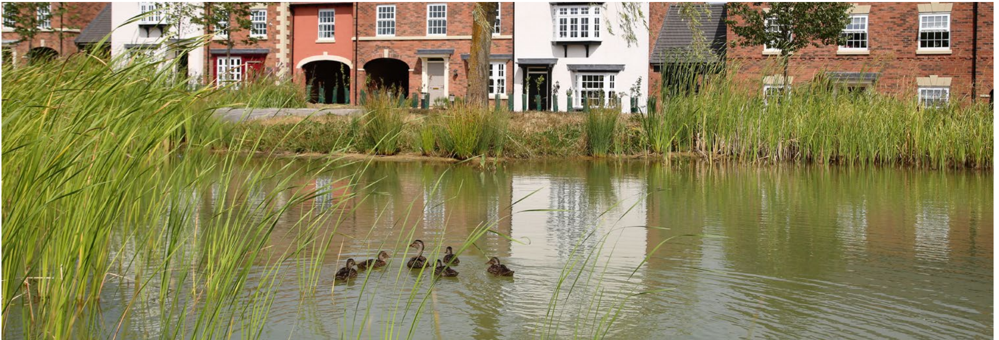
Example of sustainable urban drainage at Davidsons scheme in Houlton Rugby
