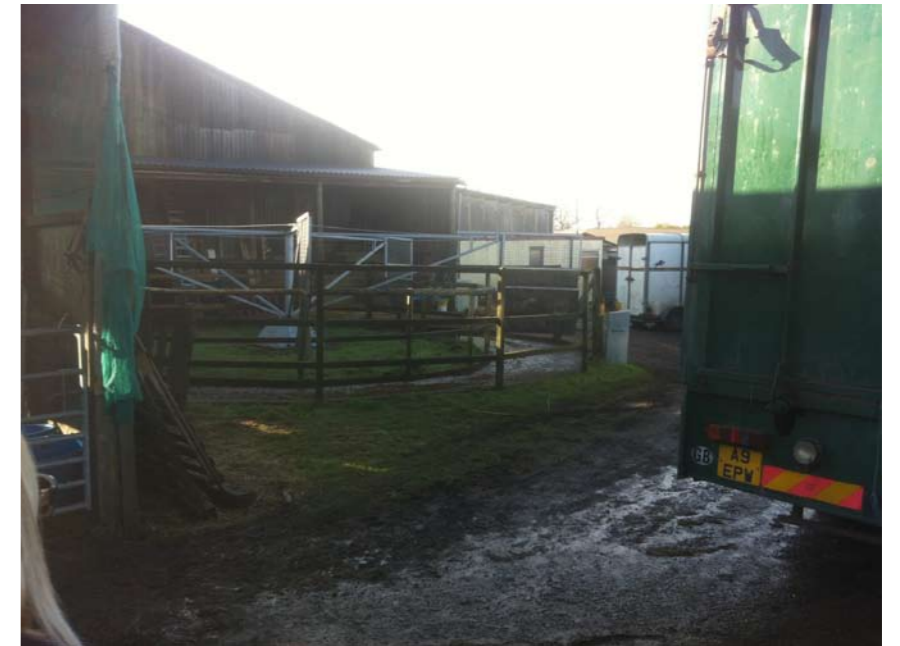
View 9 - View of horse walker and rear of large barn
