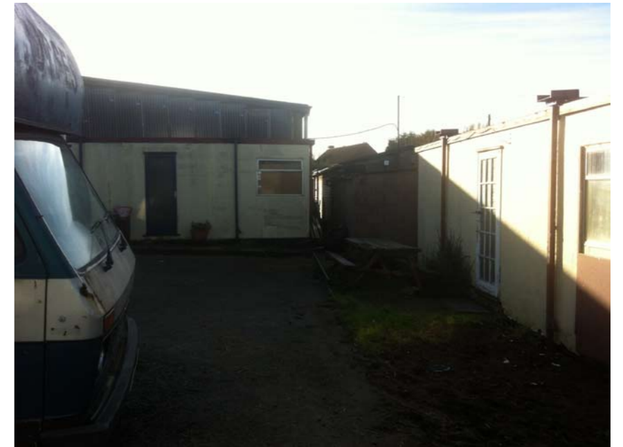
View 12 - View of rear of barn and porta cabins
