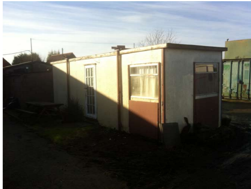
View 11 - view of porta cabins and storage containers
