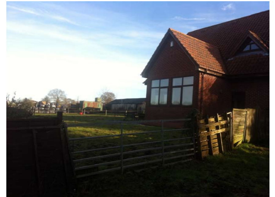
View 27 - Rear view of dwelling
