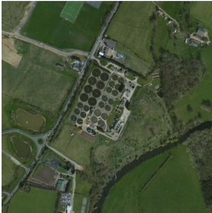
Figure 4i: Longbridge Sewage Treatment Works
