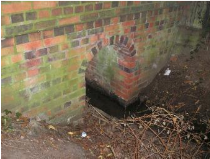
Figure 4b: Gog Brook culvert beneath A4177
