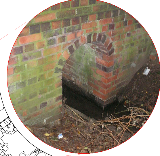
Culvert Beneath A4177
