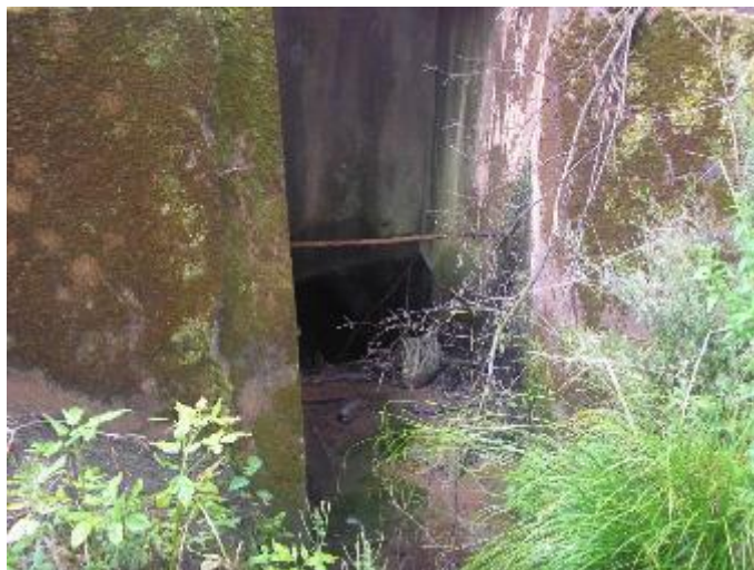
Figure 4c: Gog Brook / Grand Union Canal Culvert
