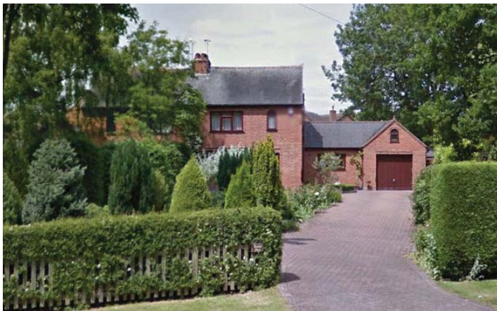
Semi-detached dwelling on Glasshouse Lane
