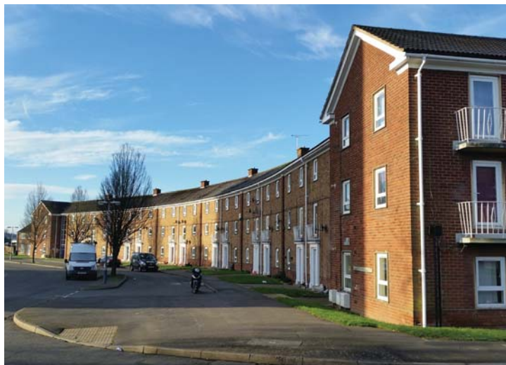
Strong block form/focal building on Newland Road
