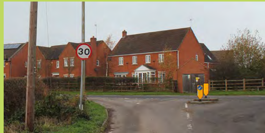
Substation on Westwood Heath Road
