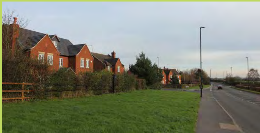
Service corridor along Westwood Heath Road
