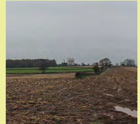
Views to Tile Hill water tower
