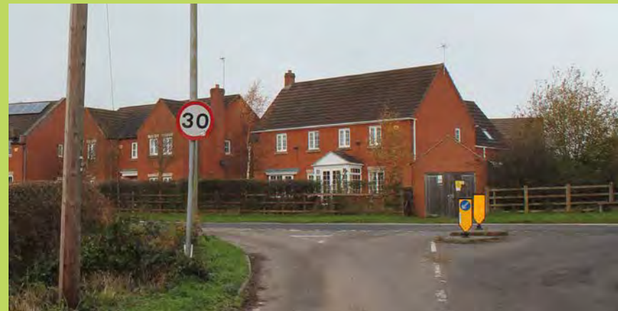
Substation on Westwood Heath Road
